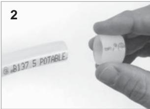
Slide ProPEX ring onto tubing
