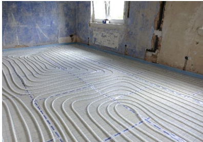
Radiant heating and cooling
