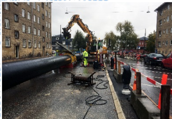
PE pressure pipes and prefabricated fittings for the Copenhagen metro: Copenhagen, Denmark
