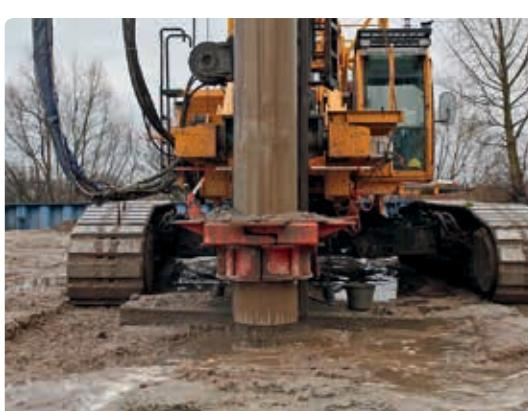
Assembly of a bore pile
