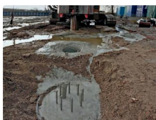
Prefabricated concrete bored pile
