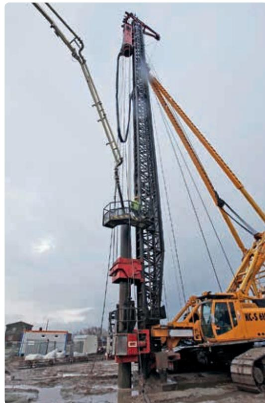
Concreting procedure of the in-situ piles
