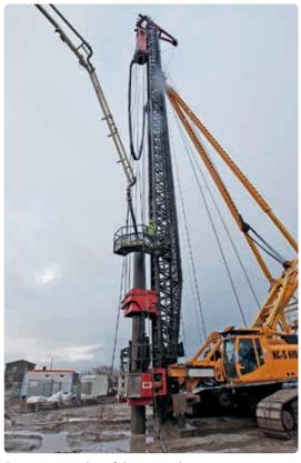
Concreting procedure of the in-situ piles
