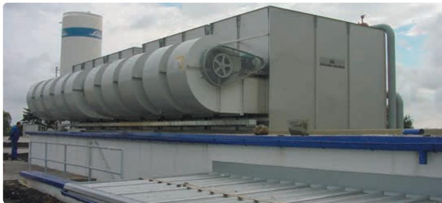
Recooling unit with pressure boosting [www.dretec.de](http://www.dretec.de)
