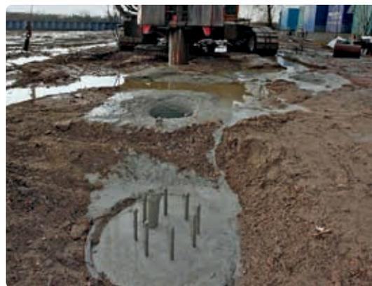
Prefabricated concrete bored pile
