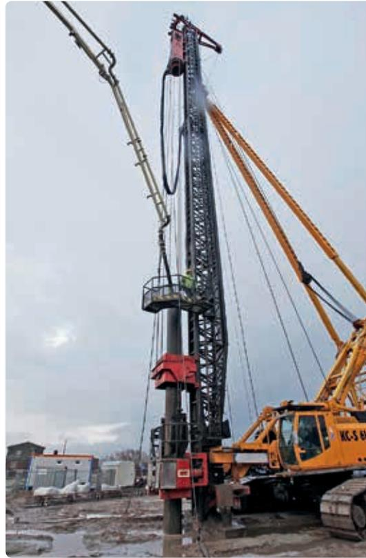
Concreting procedure of the in-situ piles
