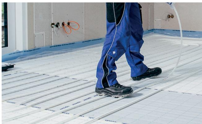
The intermediate spaces are filled with Uponor KLETT panels and the underfloor heating pipe is laid quickly and easily over the entire area of the room.
