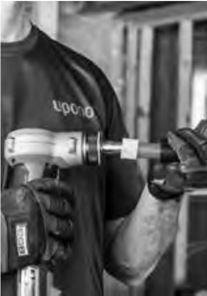
Figure 3-5: Making a ProPEX connection
