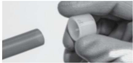
Figure 3-7: Place ring on pipe
