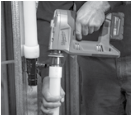
Figure 3-13: Milwaukee M18 ProPEX expansion tool
