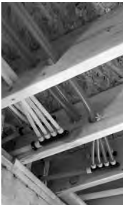
Figure 5-7: Bundled Uponor AquaPEX pipe
