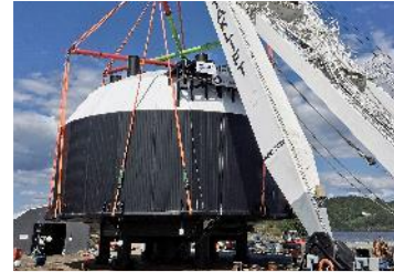
Strong and durable floating fish farming facility to withstand the harsh conditions of the Norwegian Sea Stavanger, Norway
