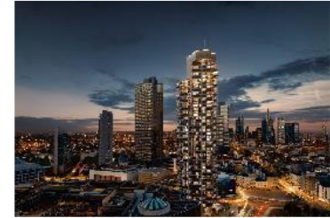
Decentralised heating and cooling for the tallest residential building in Germany Grand Tower, Frankfurt, Germany
