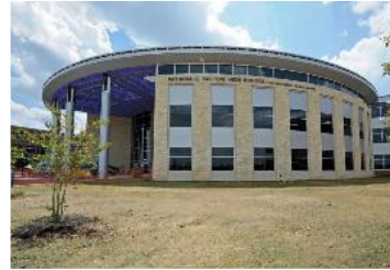
Texas high schools switch to PEX plumbing system Texas, USA
