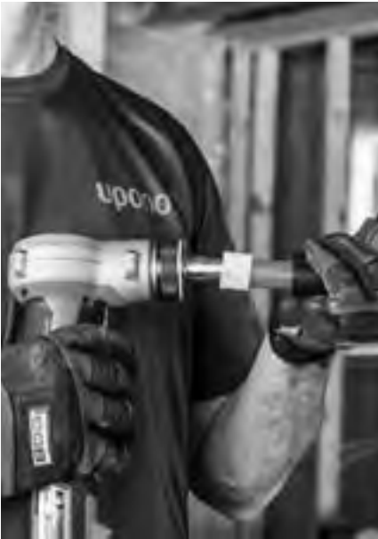
Figure 3-5: Making a ProPEX connection
