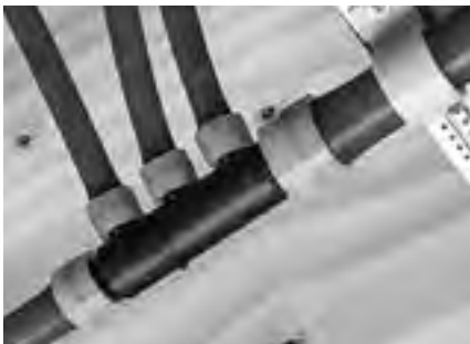
Figure 5-9: Multiport tee installation
