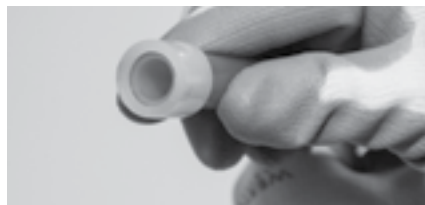
Figure 3-8: Ensure pipe reaches ring's stop edge
