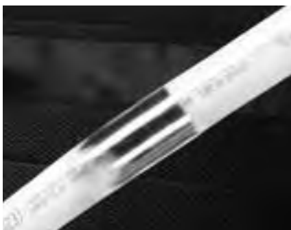
Figure C-1: Reforming kinked piping
