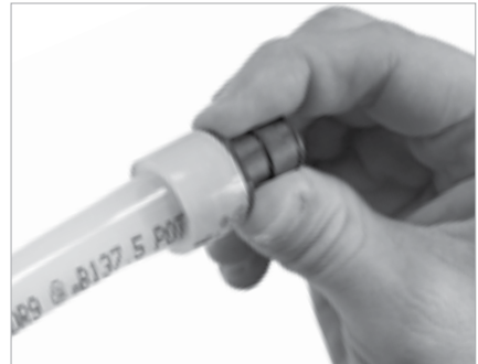
Figure 3-14: Insert the fitting
