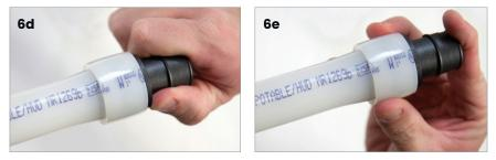
Figure 4-7: Inserting ProPEX fitting into 1" Uponor PEX piping
