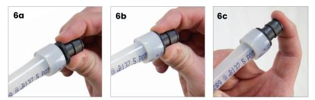
Figure 4-6: Inserting ProPEX fitting into ½" Uponor PEX piping
