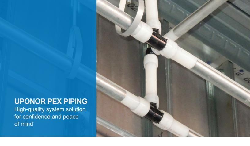
Uponor first introduced the world to crosslinked polyethylene (PEX) pipe in the early 1970s. PEX is an acronym for crosslinked polyethylene across its molecular chains.
