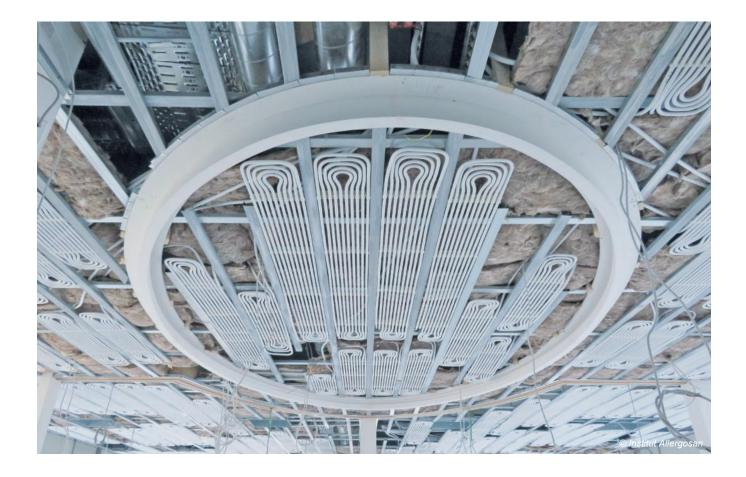
Uponor Thermatop M is a water-based heating and cooling ceiling system that operates primarily according to the radiation principle and is characterised by a variety of application and design options.
