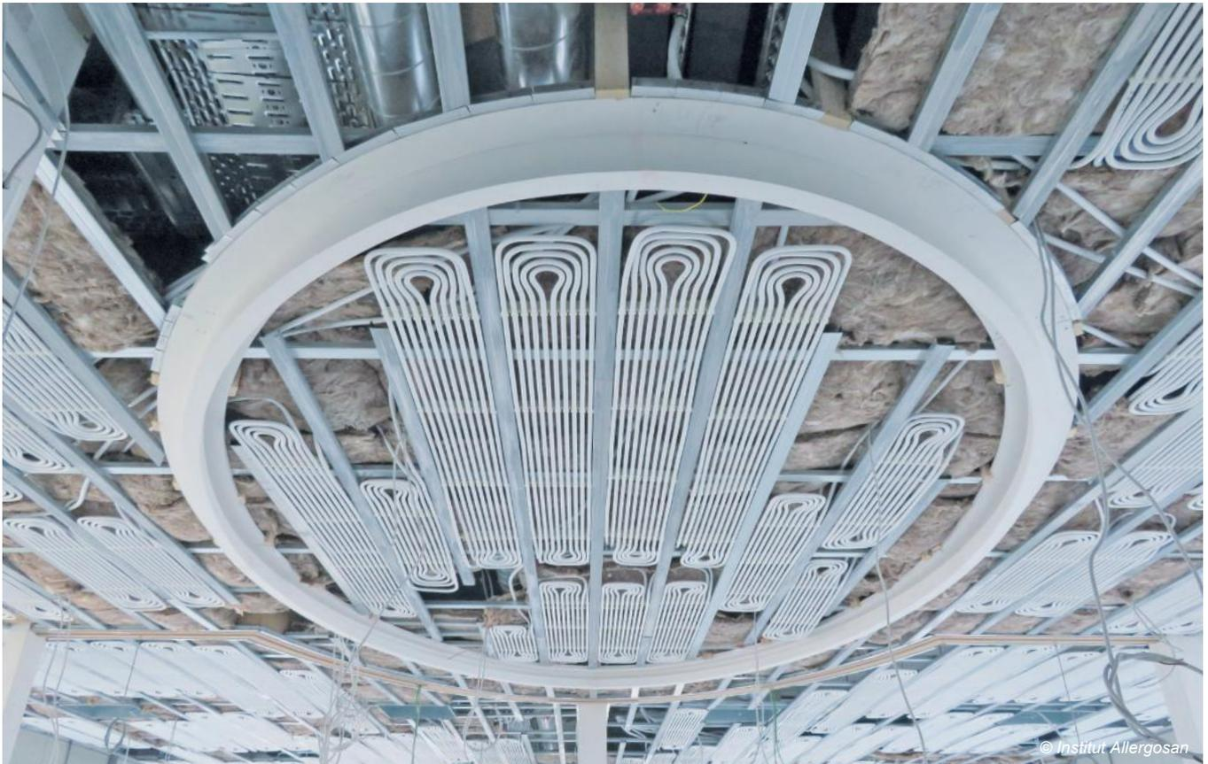
Uponor Thermanop M is a water-based heating and cooling ceiling system that operates primarily according to the radiation principle and is characterised by a variety of application and design options.
