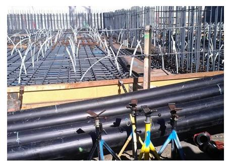
The lighter weight of PEX made it easier to move around the jobsite and its extreme flexibility made it fast and easy to install around the rebar in the base of the structure.
