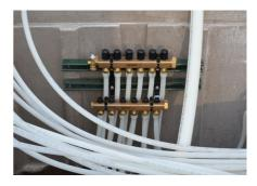
By using large-dimension tubing to feed all the manifolds, we were able to route the system efficiently and correctly.
