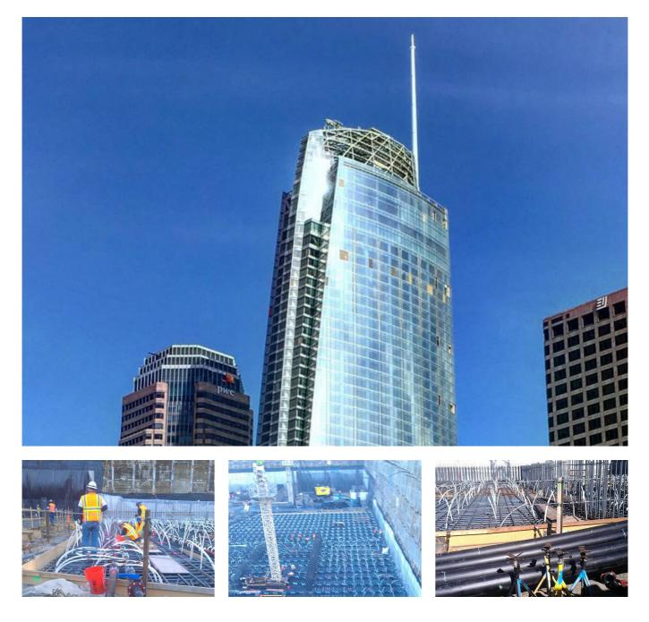
The lighter weight of PEX made it easier to move around the jobsite and its extreme flexibility made it fast and easy to install around the rebar in the base of the structure.
