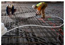
We couldn't insulate the first floor in the dowel areas, so we ended up with this checkerboard of two-inch, rigid insulation covering roughly half to 60% of the area. This checkerboard wasn't particularly easy for the installers to walk on — let alone work on — and that added to the installation time.
