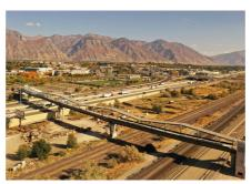
The structure is intended to move as much as 18 inches and in every direction all the time: left to right, backwards and forwards, up and down.
