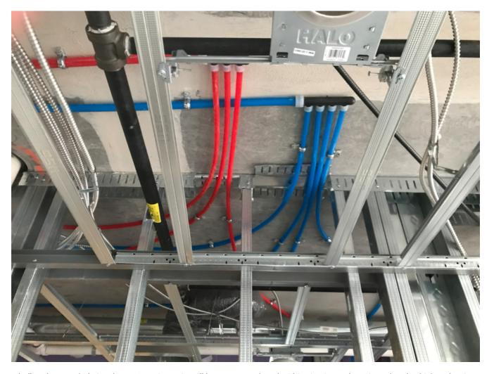
bulky, sharp-ended pipe that we're trying to install between metal studs. This pipe is much easier to bend, which makes it work for us in this project," said Thornhill. It also made long days on the jobsite easier because of its lightweight qualities that were not only forgiving on the installers' bodies, but easier to transport to the residential units situated high above the ground.
