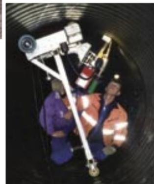
The individual pipe sections, each 12 metres in length and 1,500 mm in diameter, were assembled using an extrusion welding technique, carried out inside the pipe. The picture shows the extruder, which is mounted on a specially constructed carriage.
