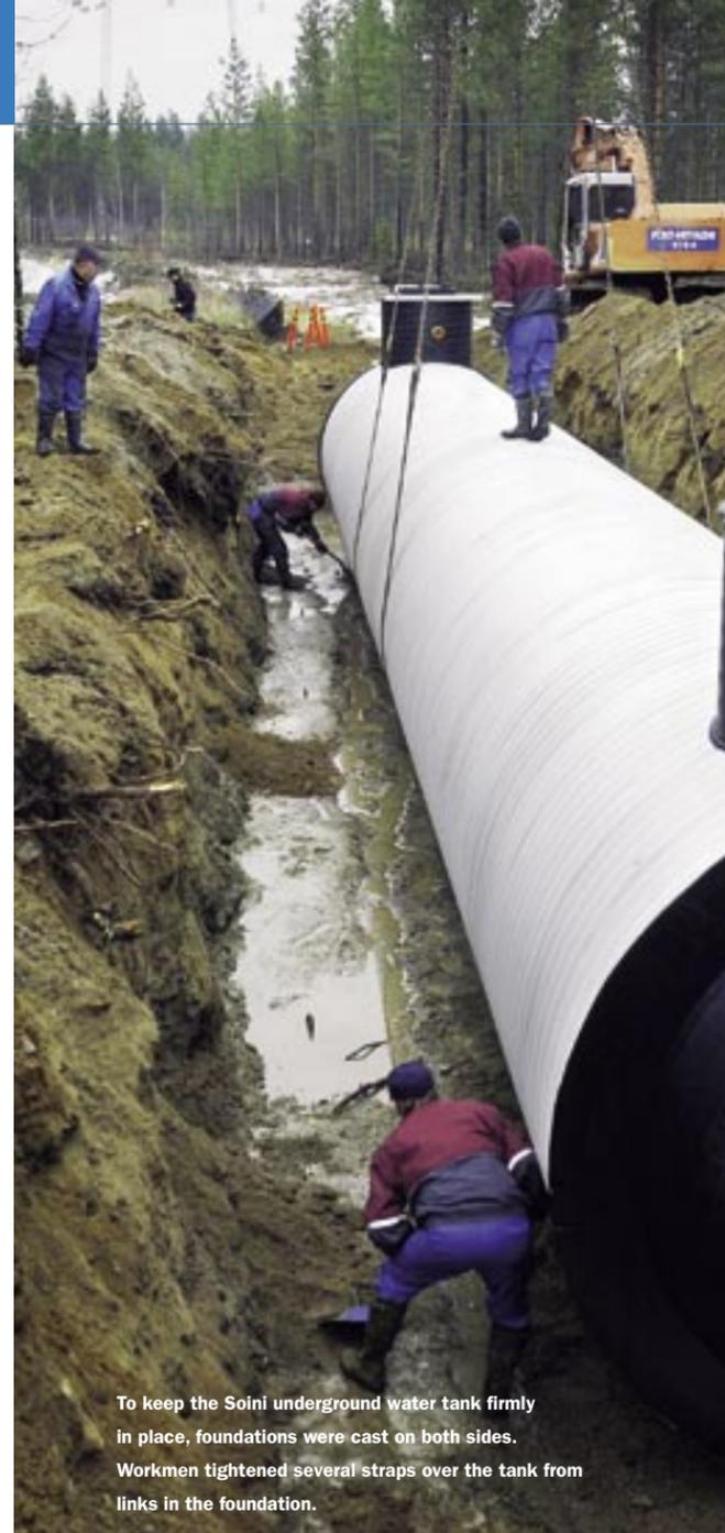
To keep the Soini underground water tank firmly in place, foundations were cast on both sides. Workmen tightened several straps over the tank from links in the foundation.
