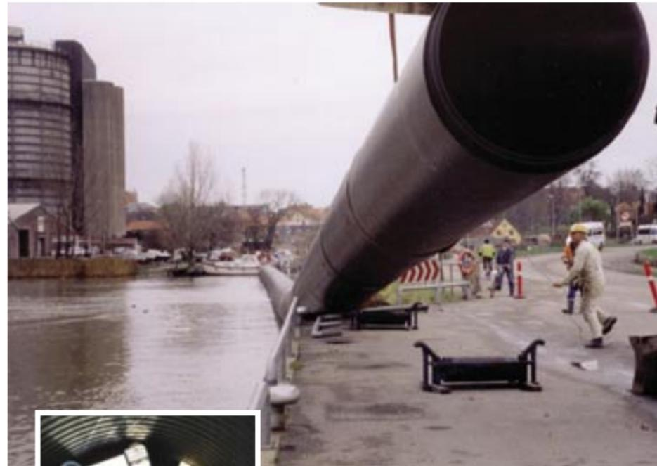
The 150-metre sewer pipe on its way into the harbour for transportation to the installation site. Note the flexibility of the pipe as it bends.
