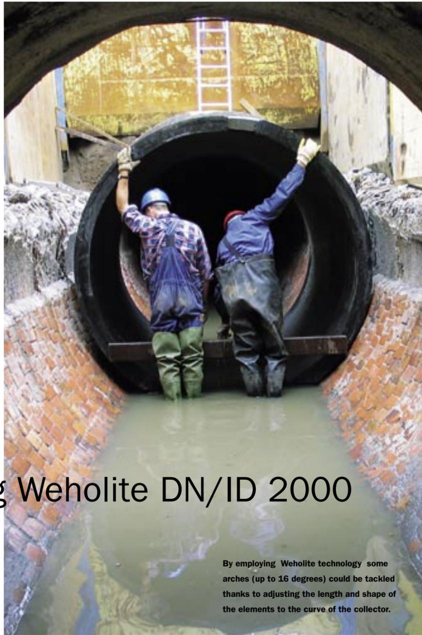
By employing Weholite technology some arches (up to 16 degrees) could be tackled thanks to adjusting the length and shape of the elements to the curve of the collector.
