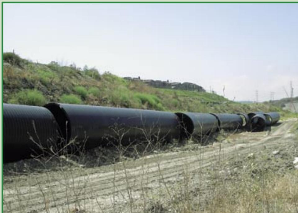
84” (2,134 mm) pipe that is strung out adjacent to where the trench was to be excavated.
