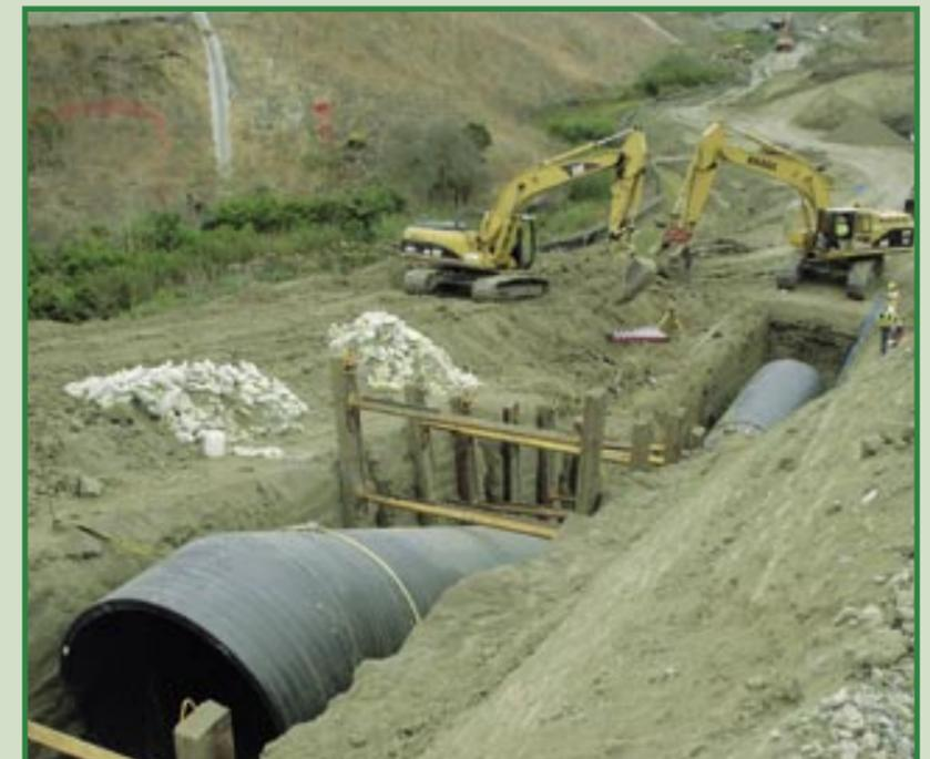
The section of 108” (2,743 mm) pipe that was constructed on a 25% grade.
