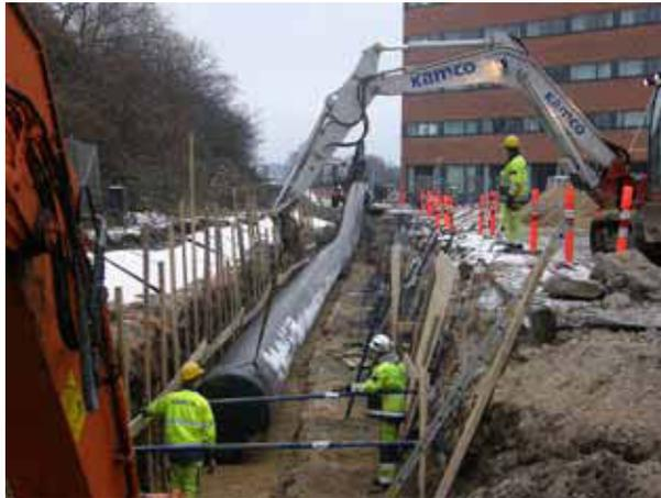
Re-laying Copenhagen's main water pipe. Shown here is the large 1,100 mm diameter pipe being laid.
