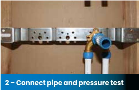
2 – Connect pipe and pressure test
