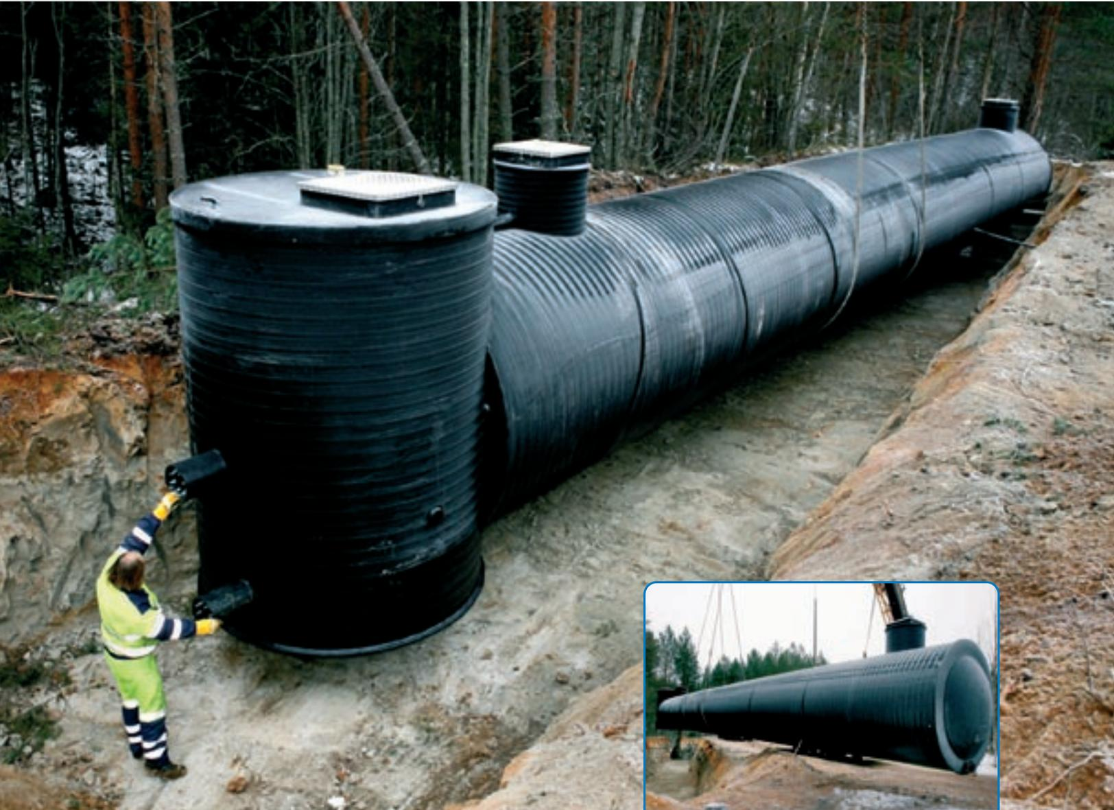
A lower-level water retention tank. The inside measurement of the Weho tank is 2,400 mm, it is 25 m long and has a volume of 100 m<sup>3</sup>. The internal diameter is 2,200 mm and the pumping chamber is attached to the end of the tank.
