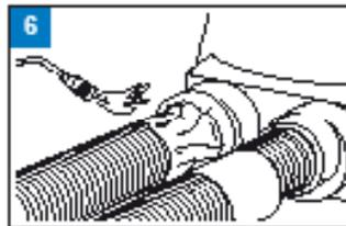
Shrink it with a soft gas flame according to the instructions on the shrink sleeve. First shrink the end near the chamber, then shrink towards the pipe element. Keep the flame in constant movement.
