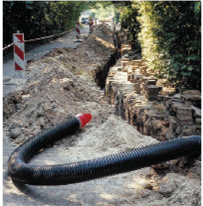
conditions, are suitable for loading by heavy traffic (SWL 60 = 60 t) according to worksheet ATV-A 127. The ring stiffness of the jacked pipe is proved according EN ISO 9969 to be able to withstand  $4 \text{ kN/m}^2$  (class SN4).
