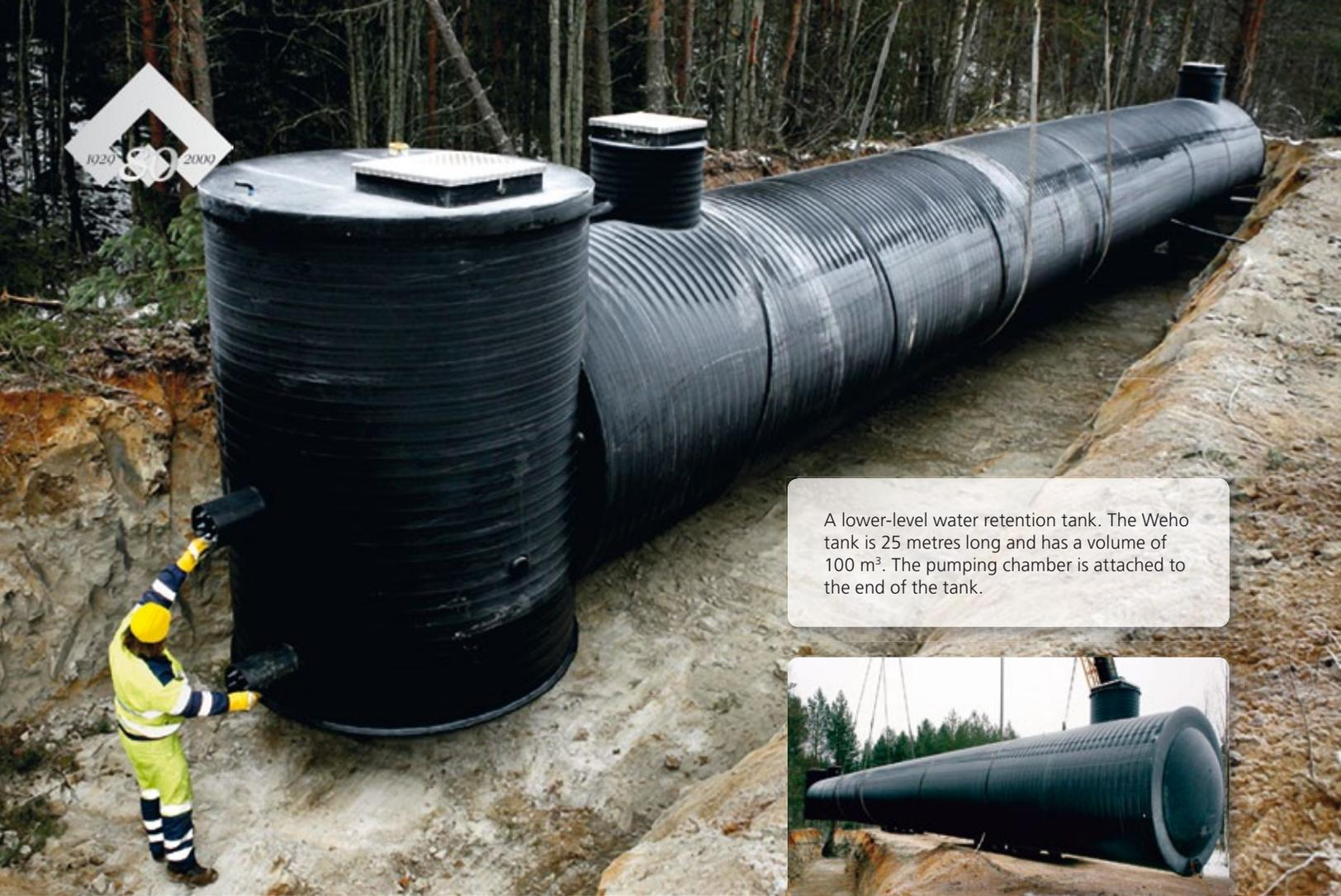
A lower-level water retention tank. The Weho tank is 25 metres long and has a volume of 100 m<sup>3</sup>. The pumping chamber is attached to the end of the tank.
