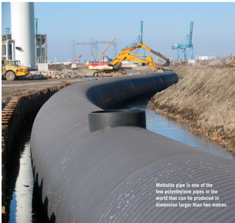
Weholite pipe is one of the few polyethylene pipes in the world that can be produced in dimension larger than two metres.
