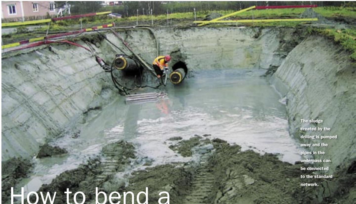
The sludge created by the drilling is pumped away and the pipes in the underpass can be connected to the standard network.
