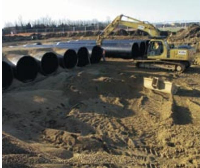
The tanks will act as a buffer between the new development and the existing main drainage system, storing storm water runoff for controlled release over time.
