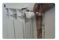
3. Fit compression adaptor to pipe and connect to valve
