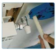
2. After test, align with radiator valve and cut back to suit
