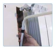
1. Connect to feed pipe and conduct system pressure test
