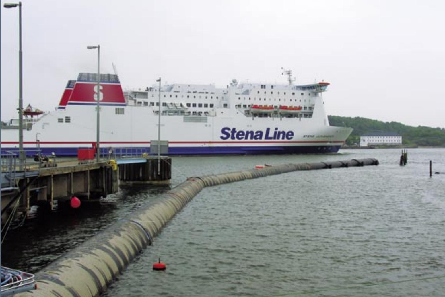
**Shipping at Sweden's busiest port, Gothenburg, was able to slip in and out of the harbour without interruption when a plastic pipeline was laid just off the harbour in May. The design was exceptional in that the pipe was weighted without external concrete weights.**
