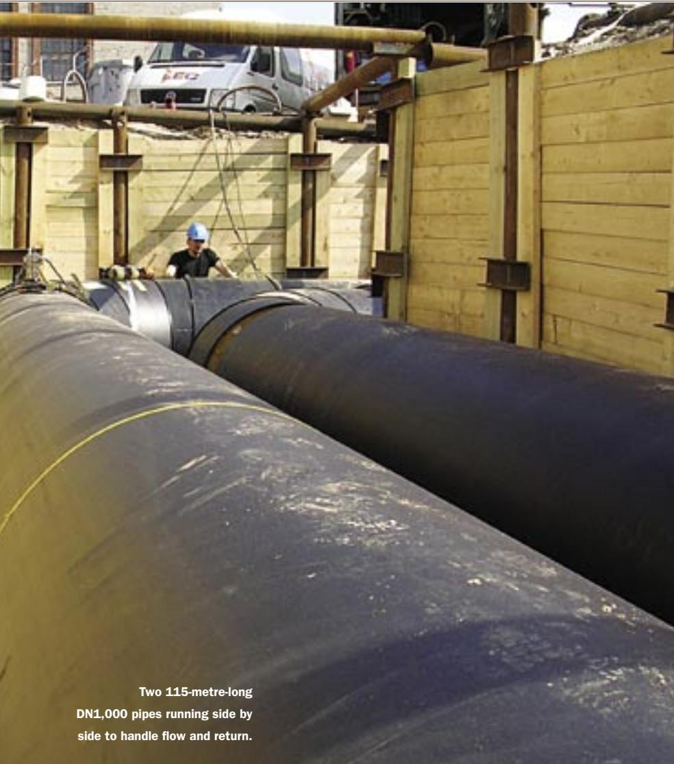
Two 115-metre-long DN1,000 pipes running side by side to handle flow and return.
