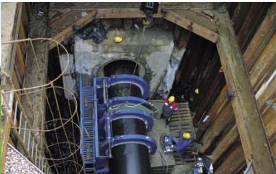
Installation of dia. 1,400 mm PE pipes in the pit under Czerniakowska St.
