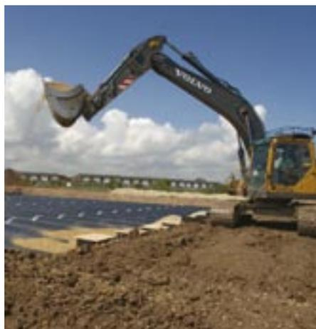
**All 15 parallel Weholite pipe runs, each measuring 2,100 mm in diameter and 114 m in length, are installed. The Weholite solution is backfilled by Seymour Civil Engineering Contractors Ltd.**
