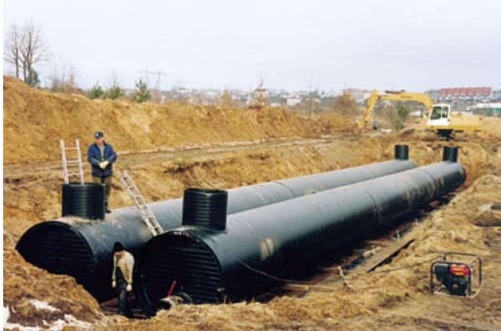
PE allow production of any manhole and fitting to order; very odd models tailor-made to optimize the properties and designs are often impossible to obtain in concrete.
