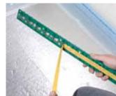
• If using Clip Rail & U-clips, lay the rail across the floor to create a matrix for the UFH pipe. Use the self -adhesive backing to hold the rail onto the insulation. For meander pattern pipe installation, set the rail out on the insulation at a maximum 500mm spacing from two opposite wall edges and a maximum 2000mm spacing between clip rails. Ensure the clip rail is at a 90° angle to the coldest external wall
