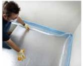
Fix the edge insulation continuously around all internal and external wall edges, using the adhesive backing. When installed correctly the PE-skirt will be facing out from the wall and the embossed 'Uponor' will be legible.
